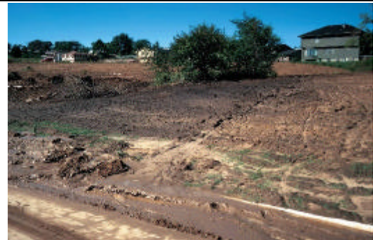
Soil erosion in a new subdivision
